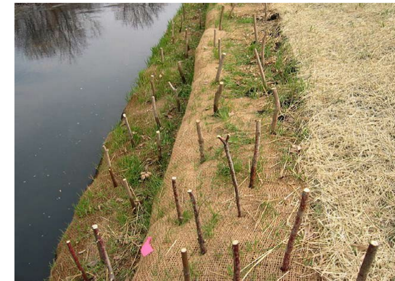
Figure 3: Live stakes along a shore 10
